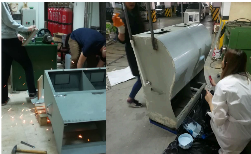
Figure 6. Team 3-Cutting steel (left) impasting weldments and coating primer (right)
